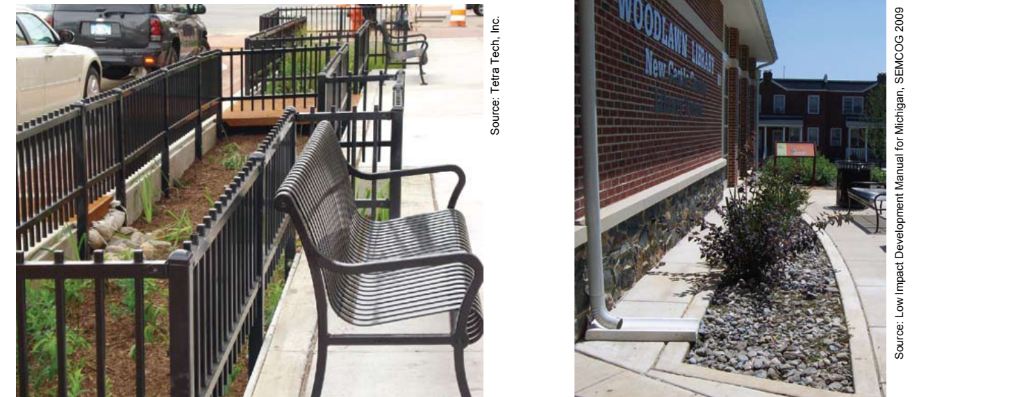
Michigan Avenue Bioretention Planter Box, Lansing, MI Example of Infiltration Planter Box
