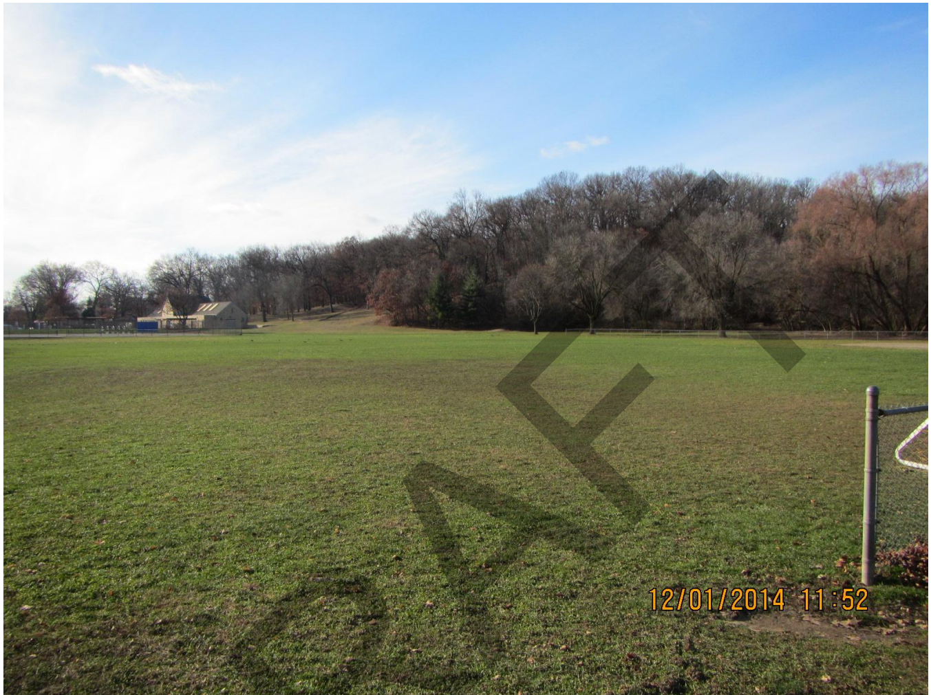
Photograph 3: General Area of 12-inch Storm Sewer under Richmond Hills Park
