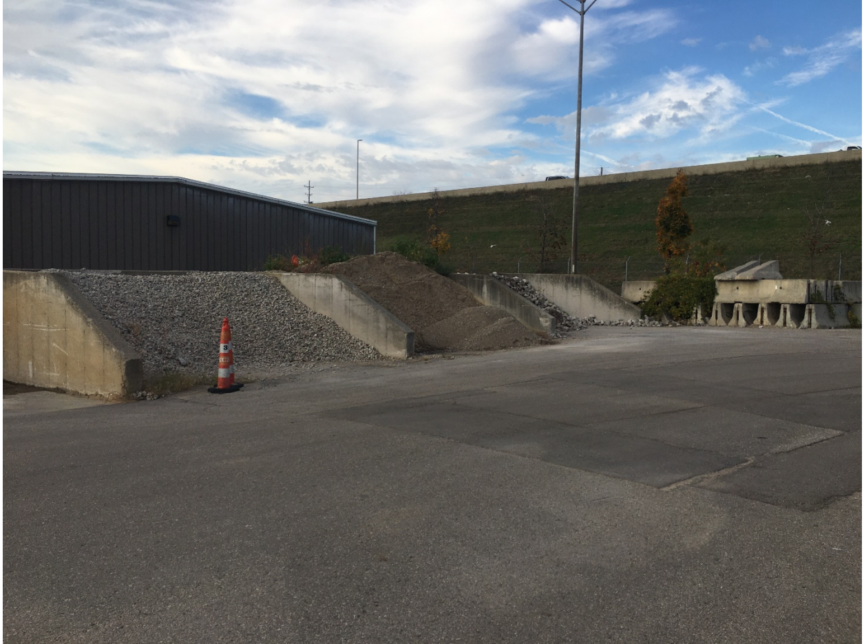
Material storage bins.
