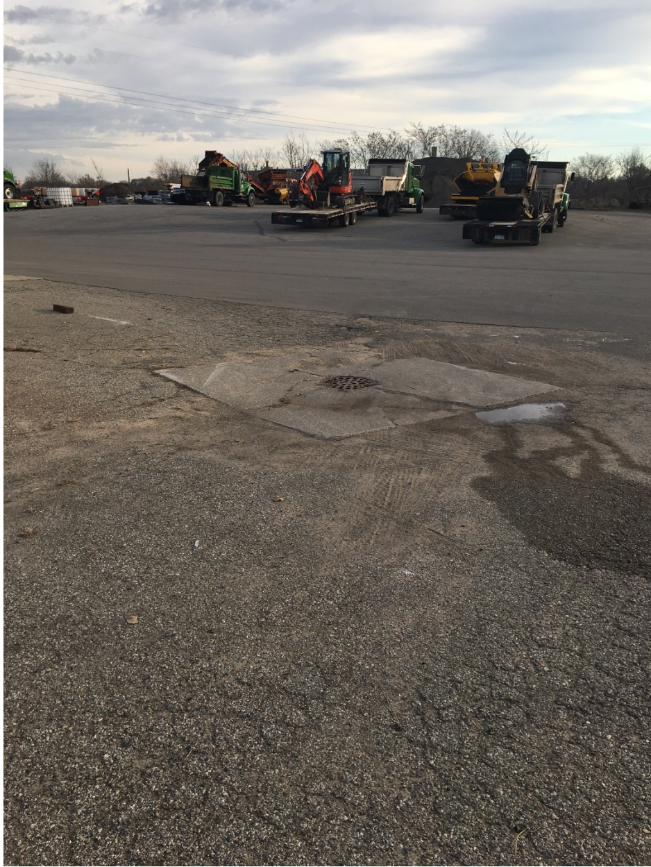
Catch basin in storage area.
