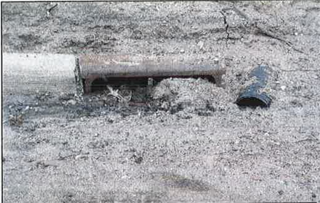
Excessive sediment from construction site.
