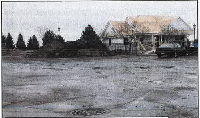
Sediment flowing into drain from soil piles.
