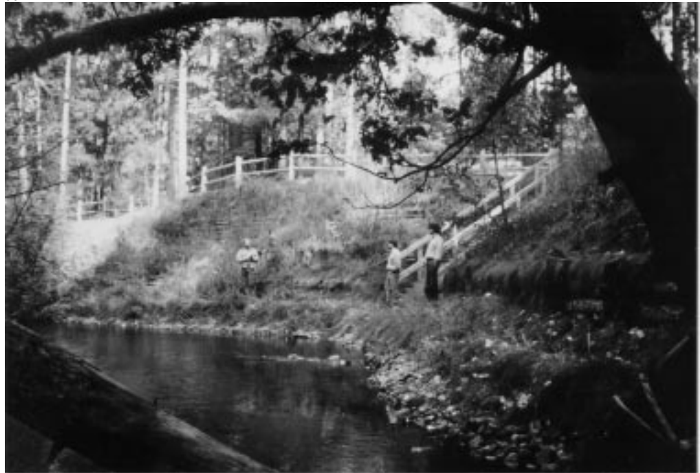
Picture 2, right: Riprap was placed to 3 feet above the ordinary high water mark and a portion back-filled with soil. Log terraces were placed on the bank and the bank
