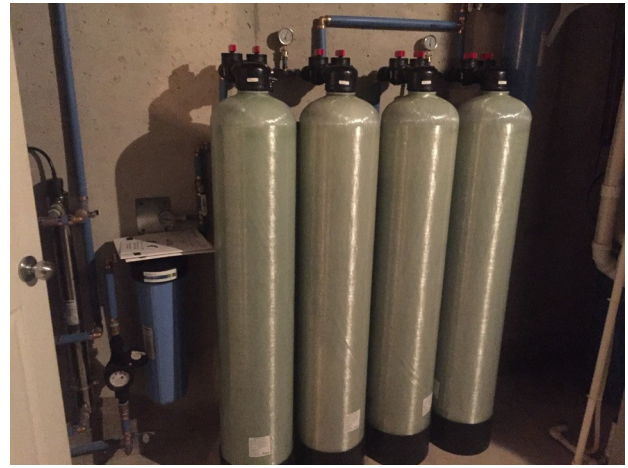
Whole-house filters like the one above have been installed in affected homes.
